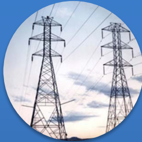
Electrical Power System and Fuel Distribution
